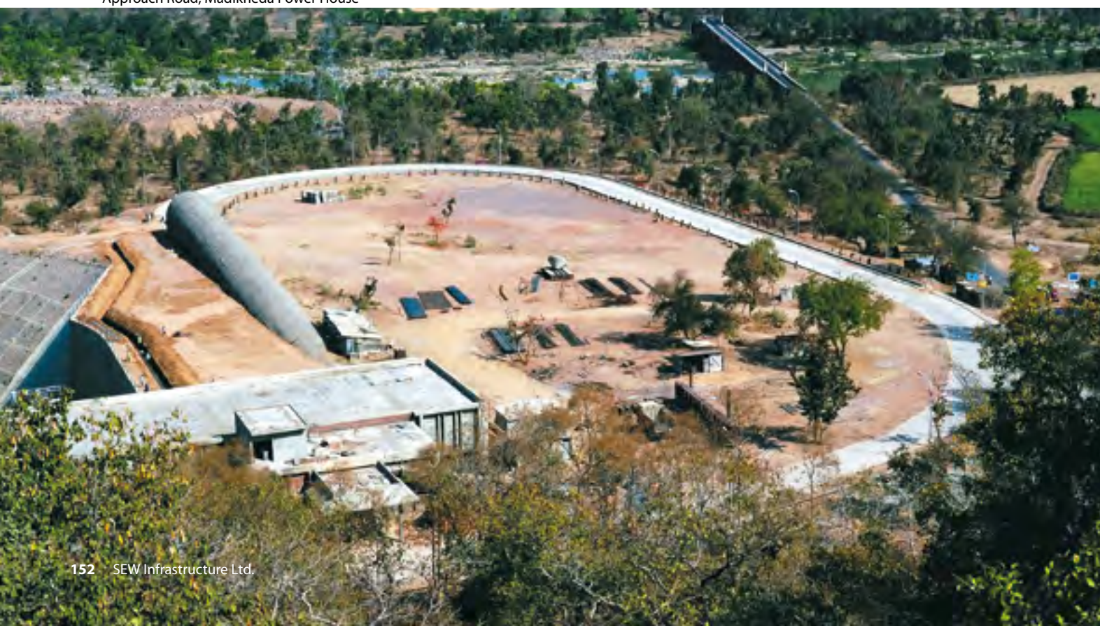
Approach Road, Madikheda Power House
