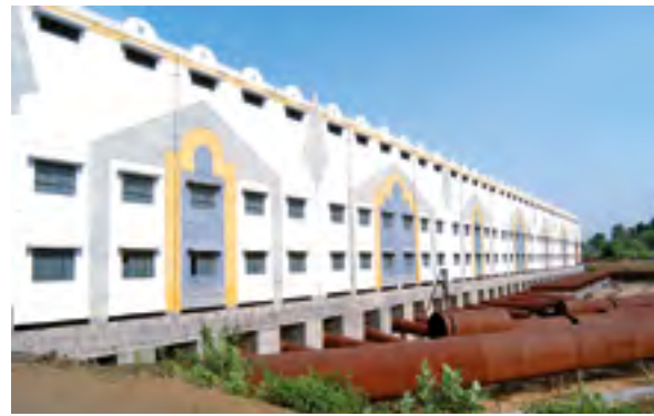
Tembhu Pump House - Discharge side
