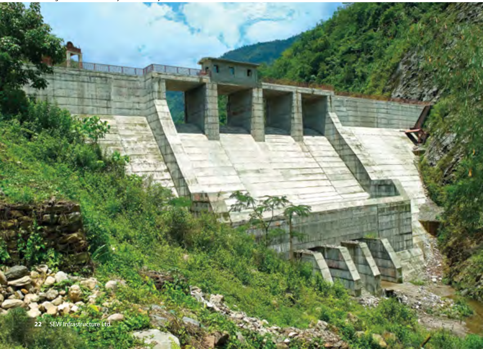
Rongli Dam - Chuzachen Hydro Power Project
