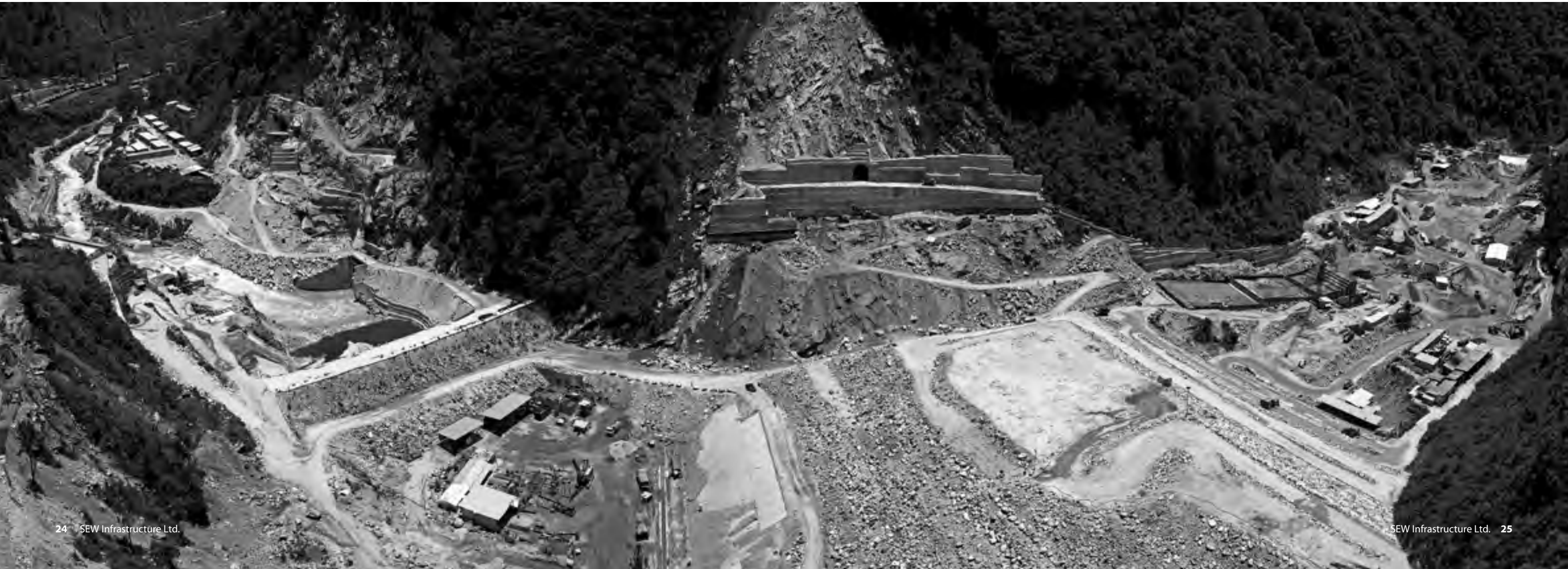
River Diversion Tunnel - Inlet, Cofferdam, Rock Filled Dam & Spillway
