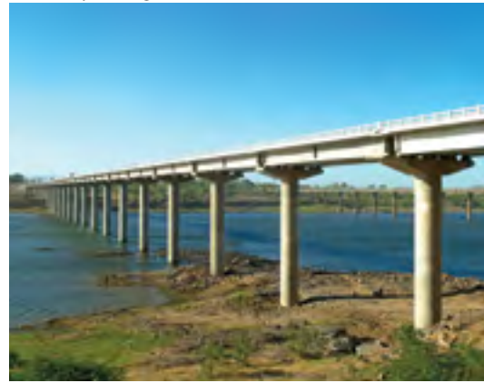
NH3 - Major Bridge
