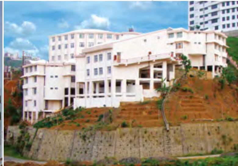
ATI Building - Rear Elevation
