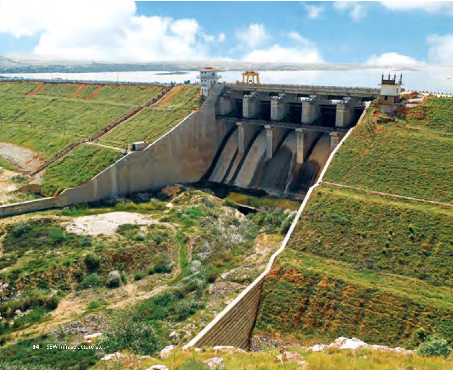
Veligallu Reservoir Dam
