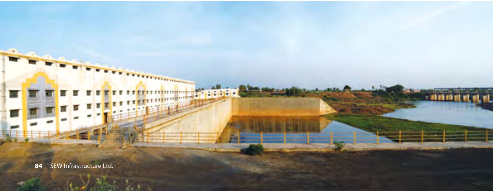
Tembhu Pump House, Barrage
