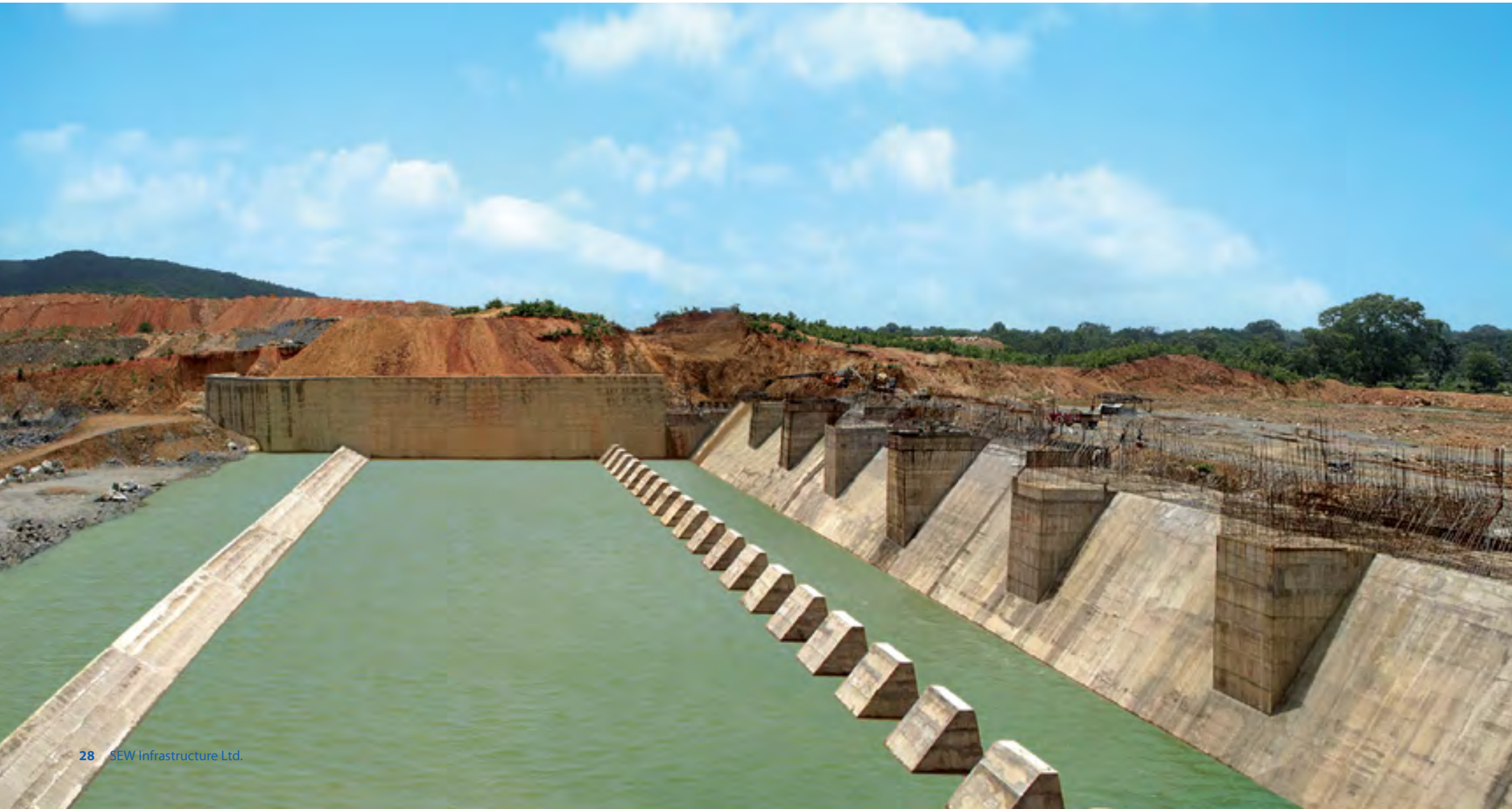
Kelo Dam, Chhattisgarh
