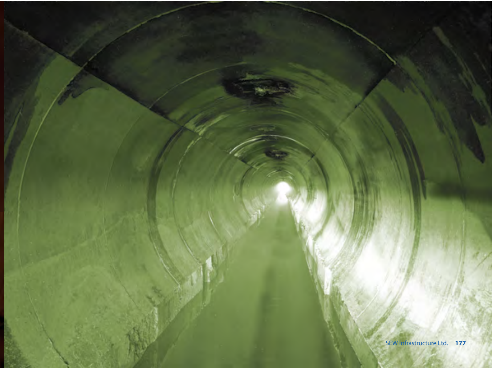
Power House Tunnel, Chuzachen HEP, Sikkim
