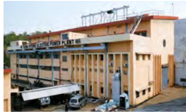
2 x 6.75 MW Tawa Power House
