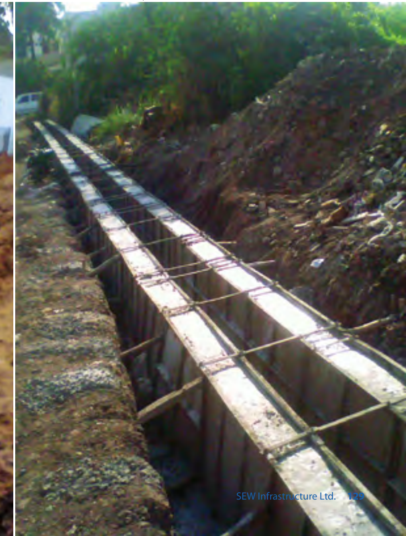
Roadside Storm Water Drains, Coimbatore CMC
