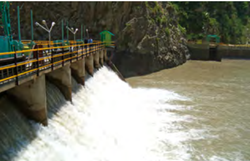
Malana Hydro Electric Project
