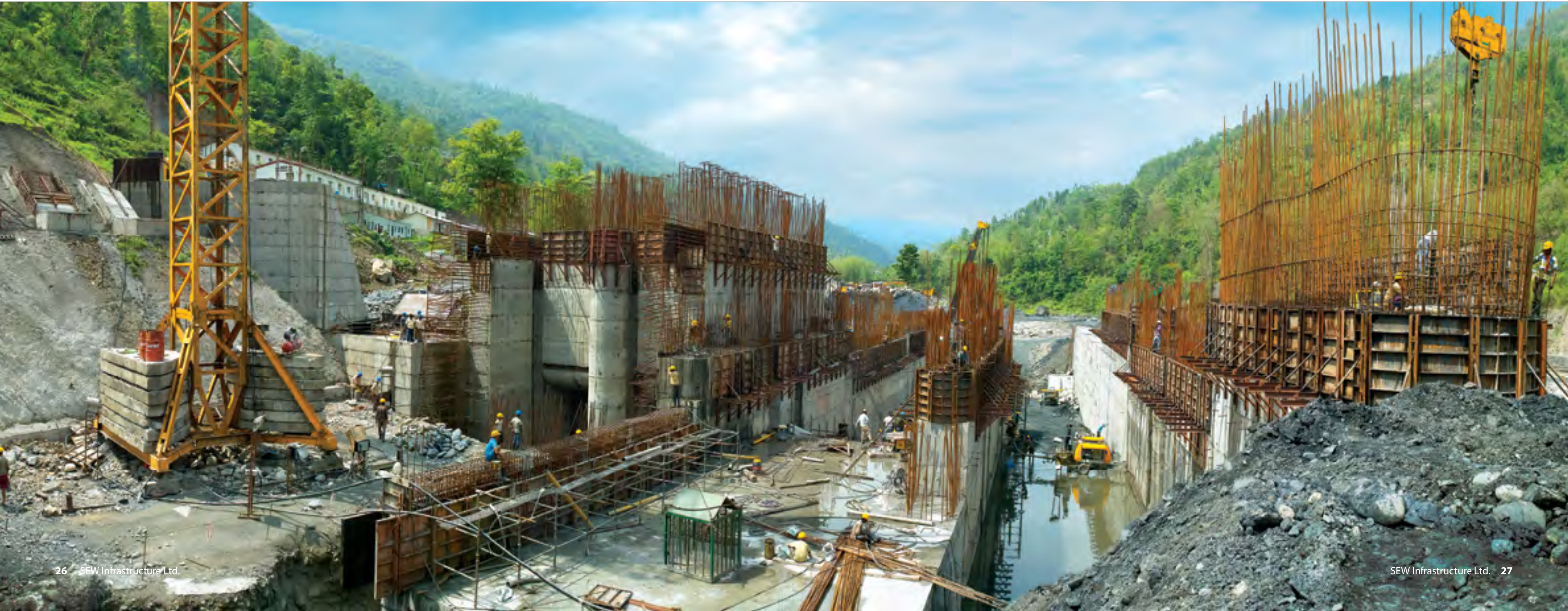
Construction of barrage for Jorethang Loop HEP
