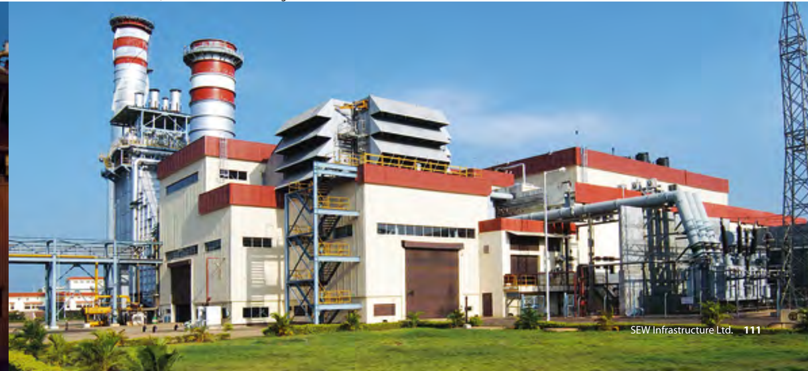
CCPP Stacks, Turbine Generator Buildings
