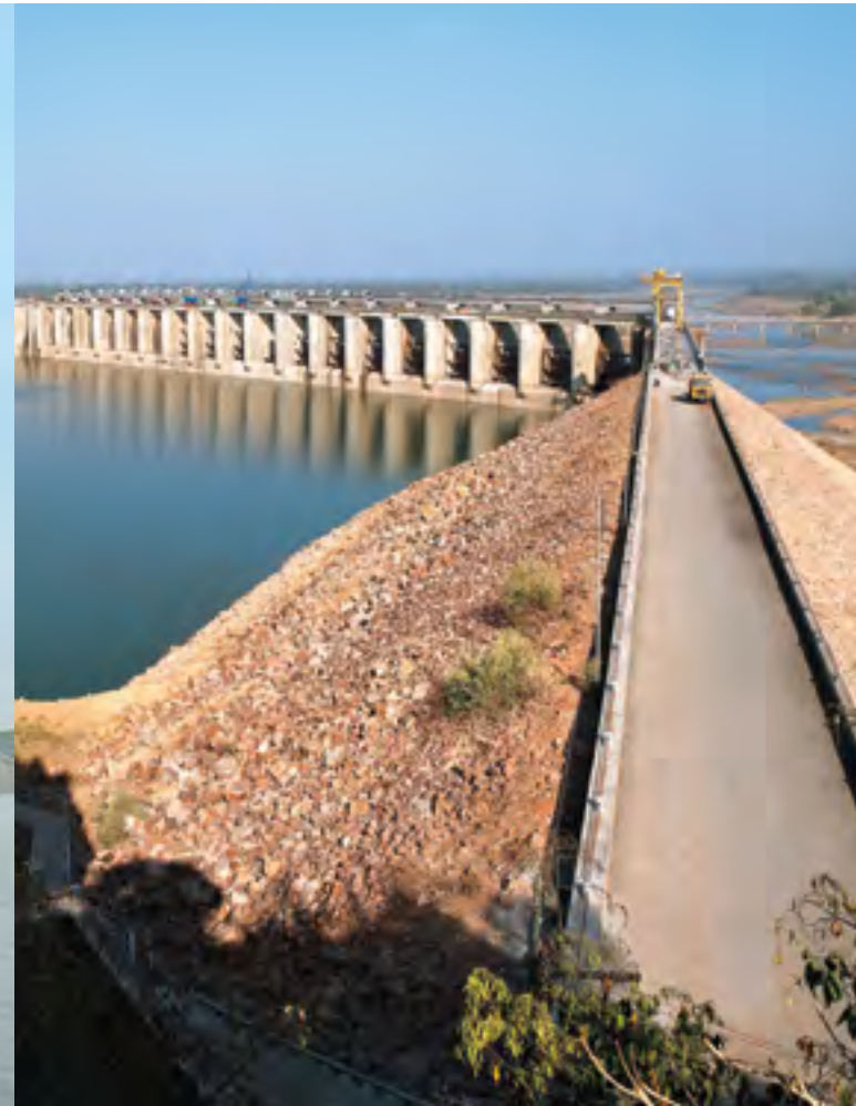
Bansagar Dam / Road Bridge
