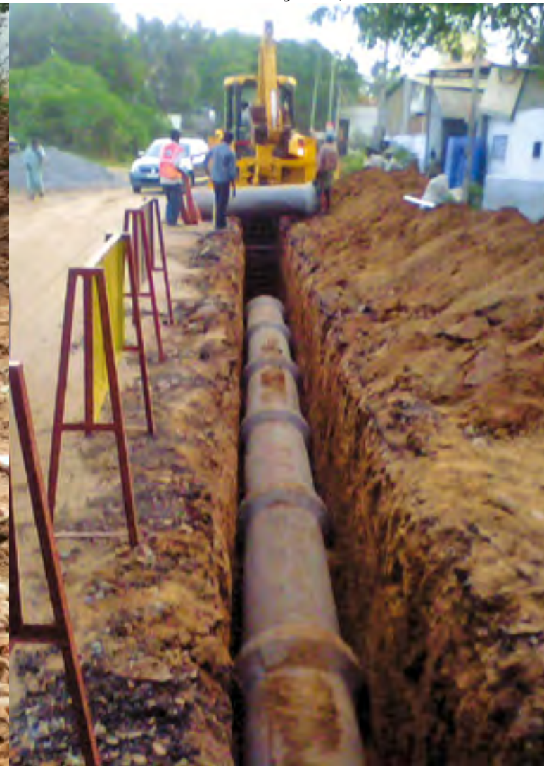
Under Ground Sewerage Works, Coimbatore CMC
