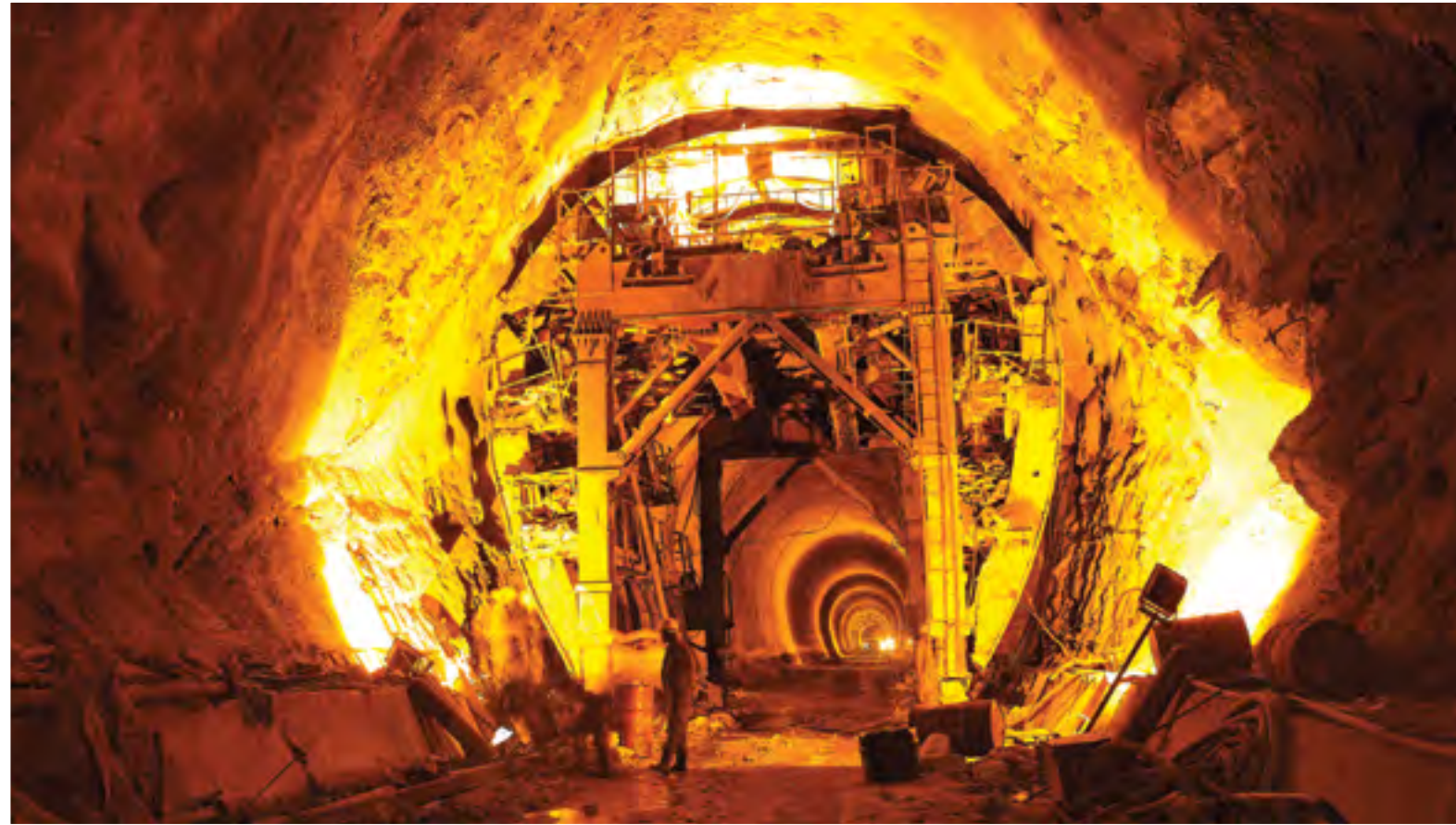
Tunnelling, Teesta III HEP
