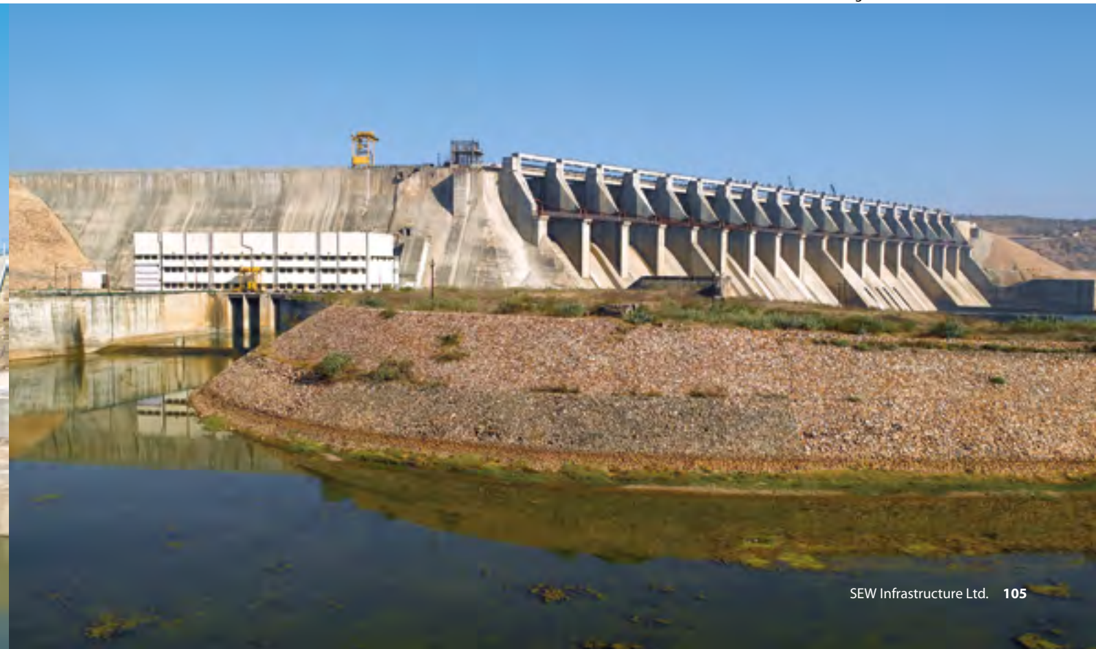
Bansagar Dam & Power House
