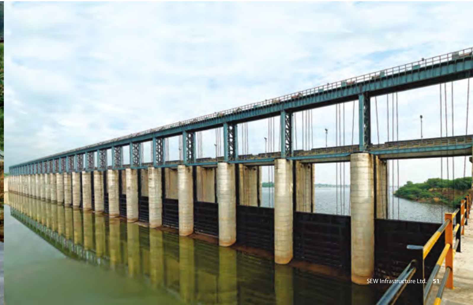
Hydro - Mechanical Works, Sulwade Barrage
