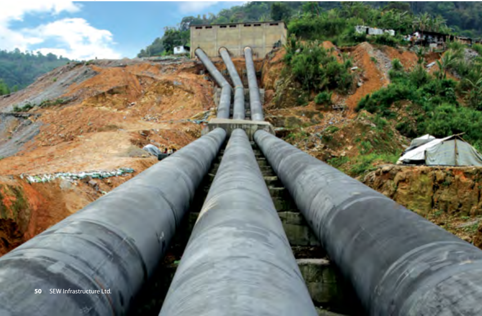
Penstock Works, Myntdu HEP
