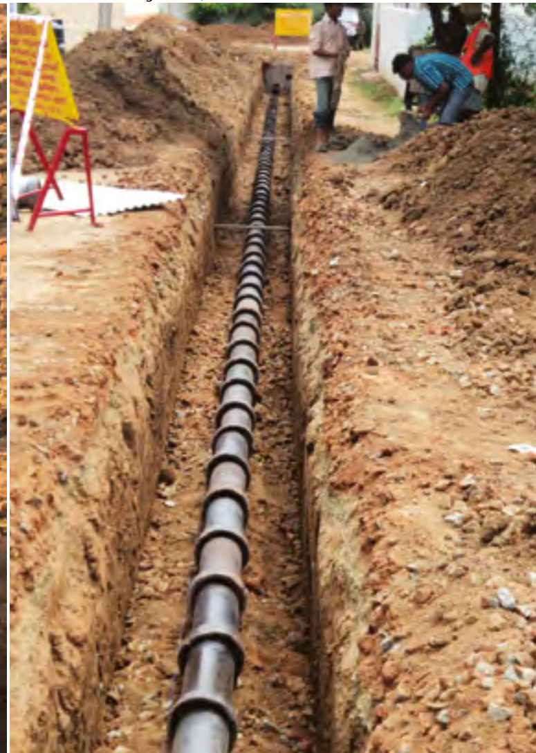
Under Ground Sewerage Works, Coimbatore CMC
