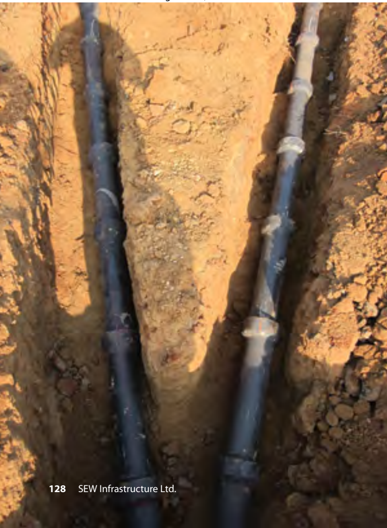
Under Ground Sewerage Works, Coimbatore CMC
