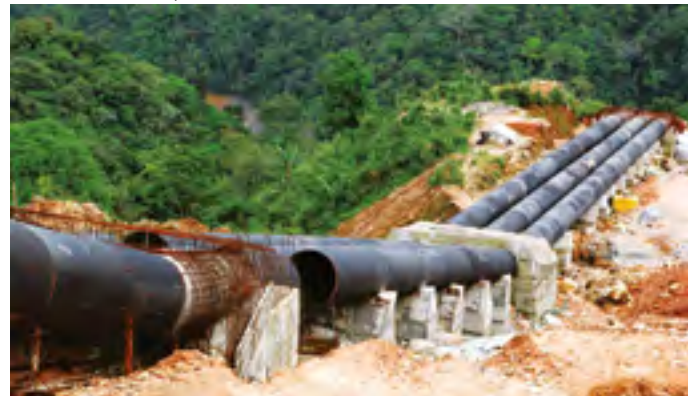
Penstock Works, Myntdu HEP
