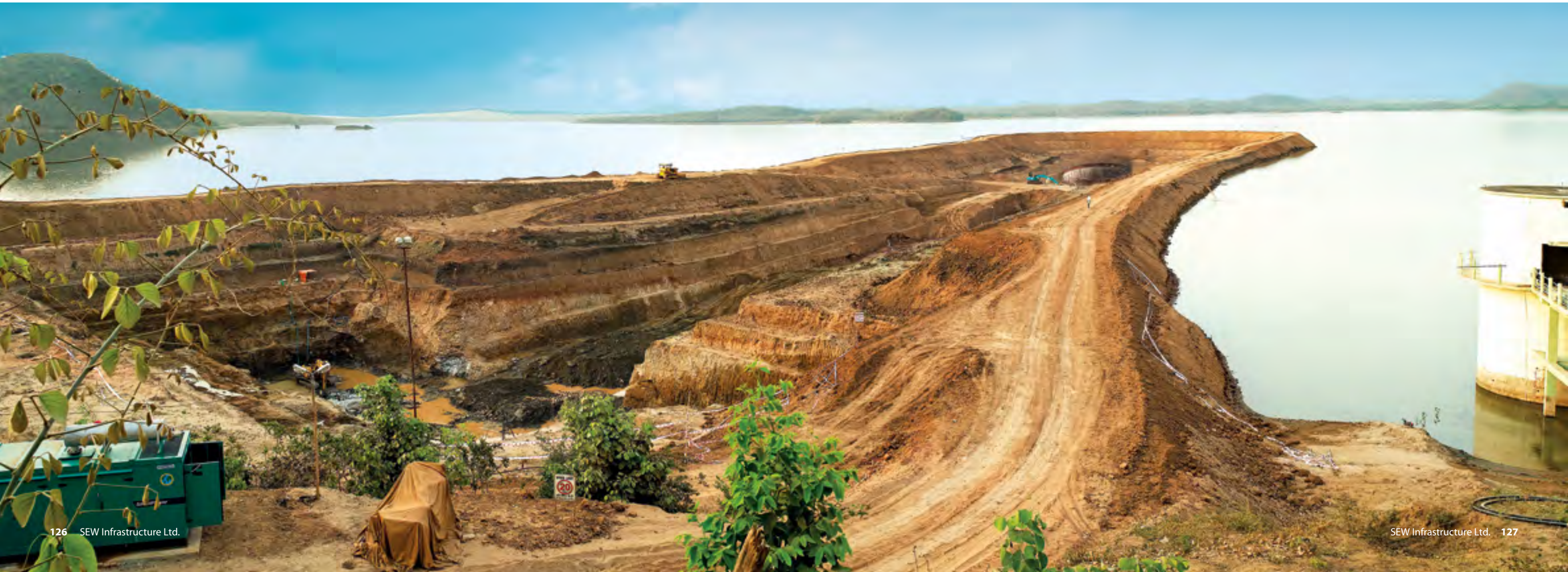
Intake Well - Panoramic View
