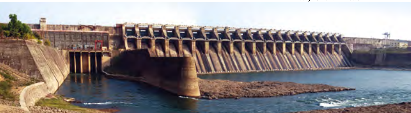
Power House, Bargi
