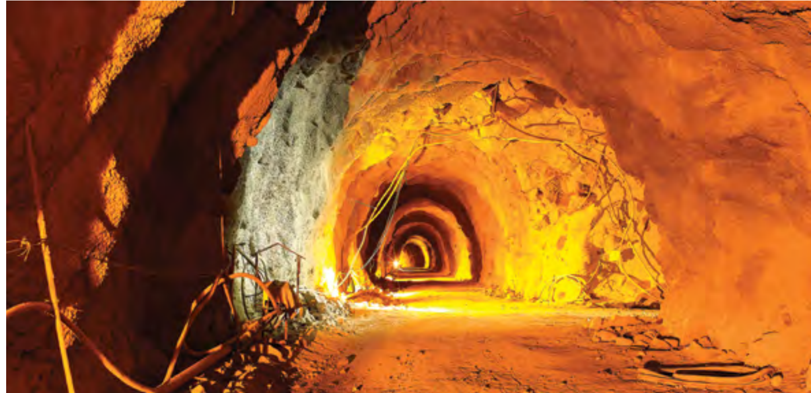
Tunnelling, Teesta III HEP
