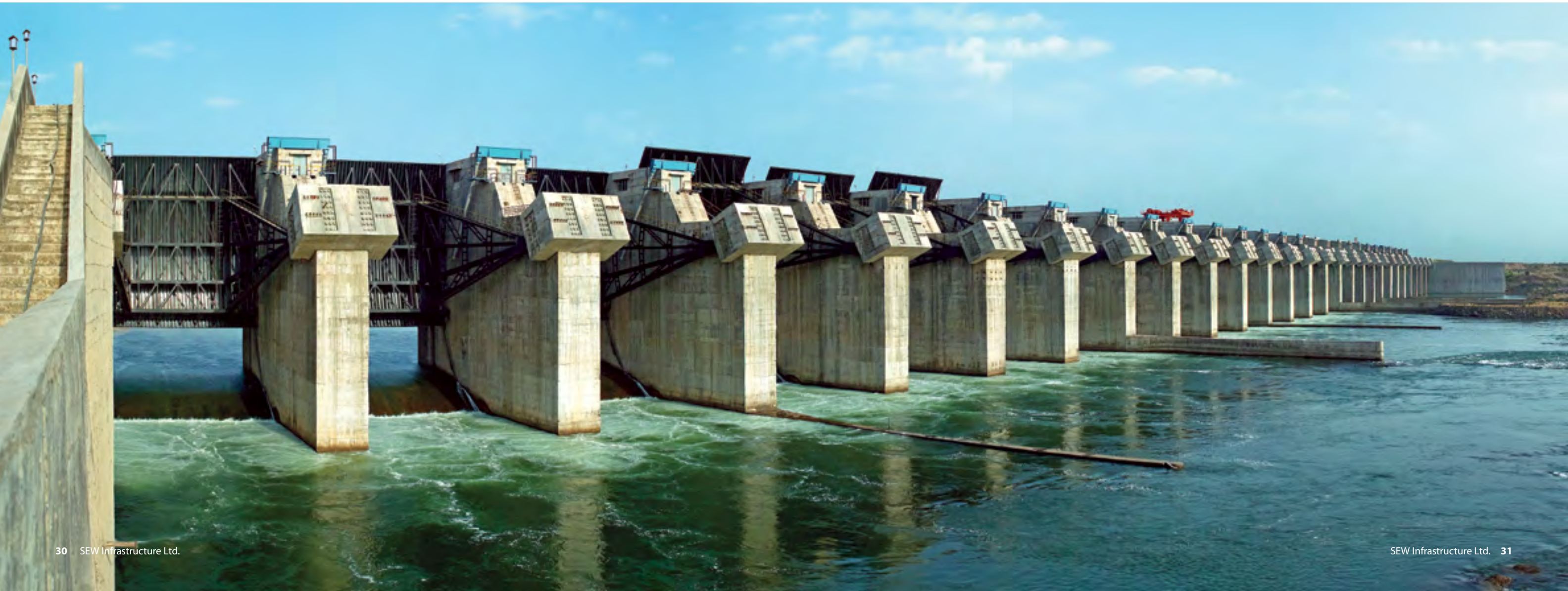
Maheshwar Dam - Downstream view
