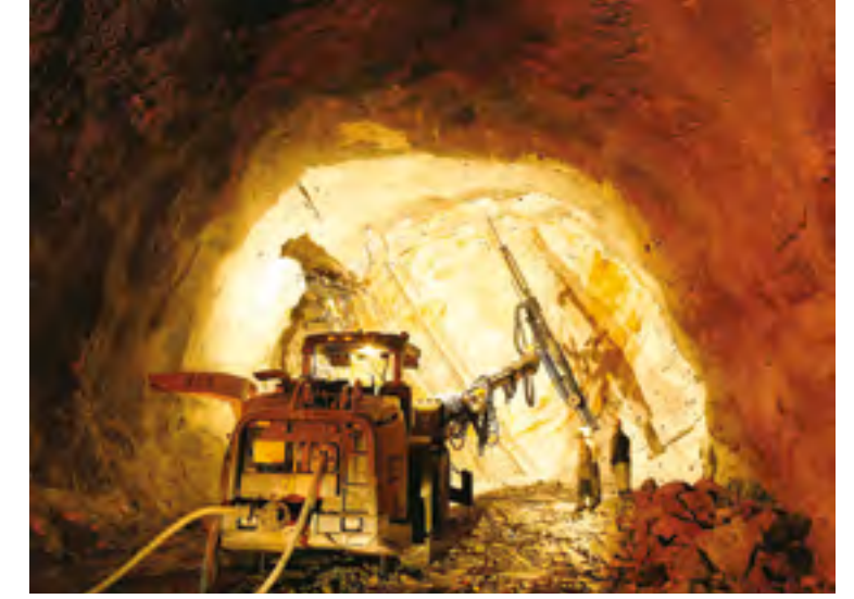
River Diversion Tunnel at Chuzachen
