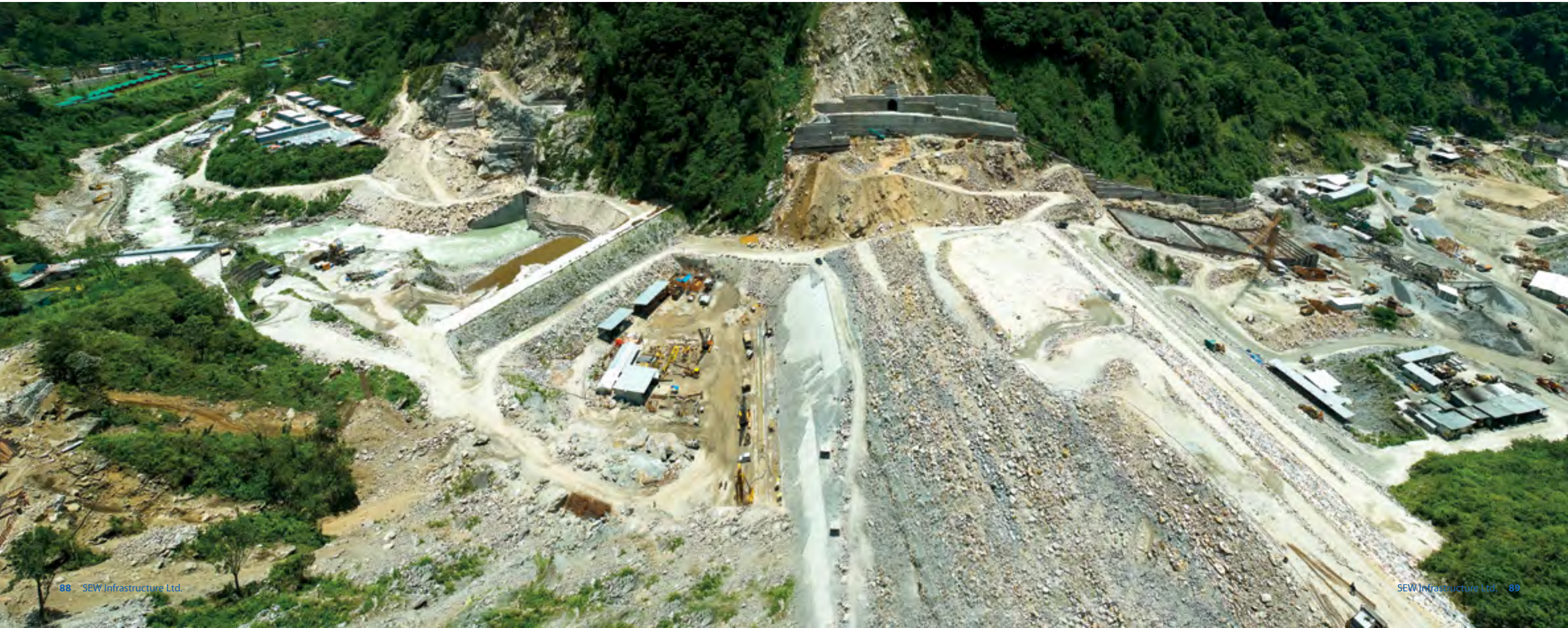
Overview of Teesta HEP - River Diversion Tunnel, Cofferdam & Rock Filled Dam
