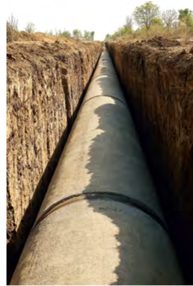
Completed Section of Pipeline
