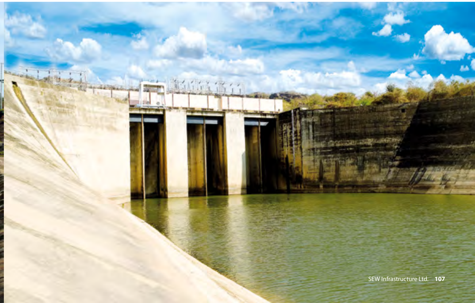
Power House Intake
