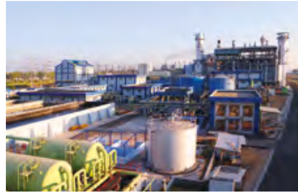
Civil Works in Transformer area
