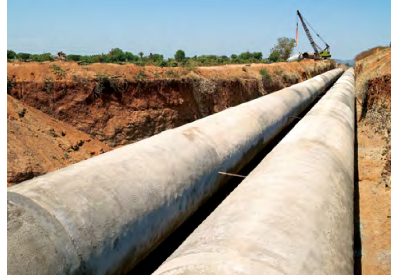
3 m dia. Pipeline Laying
