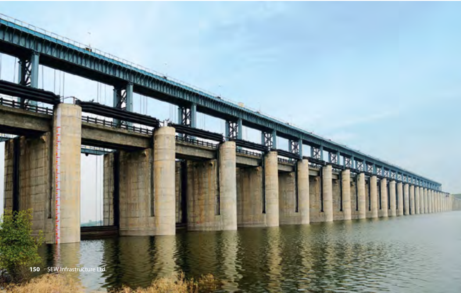
Deck Bridge, Sulwade Barrage
